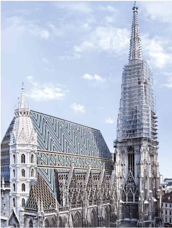
We used a bespoke modular scaffolding system for St. Stephen's Cathedral in Vienna which was erected around the building without the use of anchors
